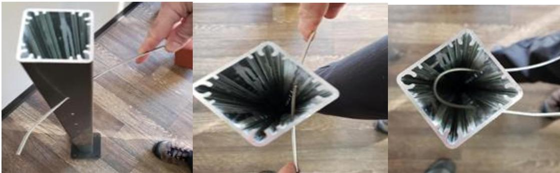
Drop the 1/2 galvanized pipe into the post through the cable loops. Once the galvanized pipe is all the way in the post, pull the cables towards you to tighten the hold with the pipe. Do this for all cables in the corner post.
