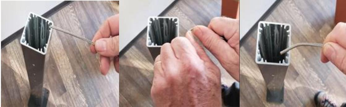
Start by inserting the bent cable through the drilled hole in the post. Then, lace the cable through the post to the corresponding drilled hole on the other side of the post. Do this for all cables. Once the cables are installed through corner post, push the cable back into post to create a loop.
